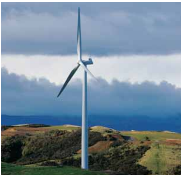
A typical horizontal axis wind turbine. This is a turbine at Te Apiti. It has a 1.65MW generator on a 70 metre high tubular steel tower with 36 metre long blades.
