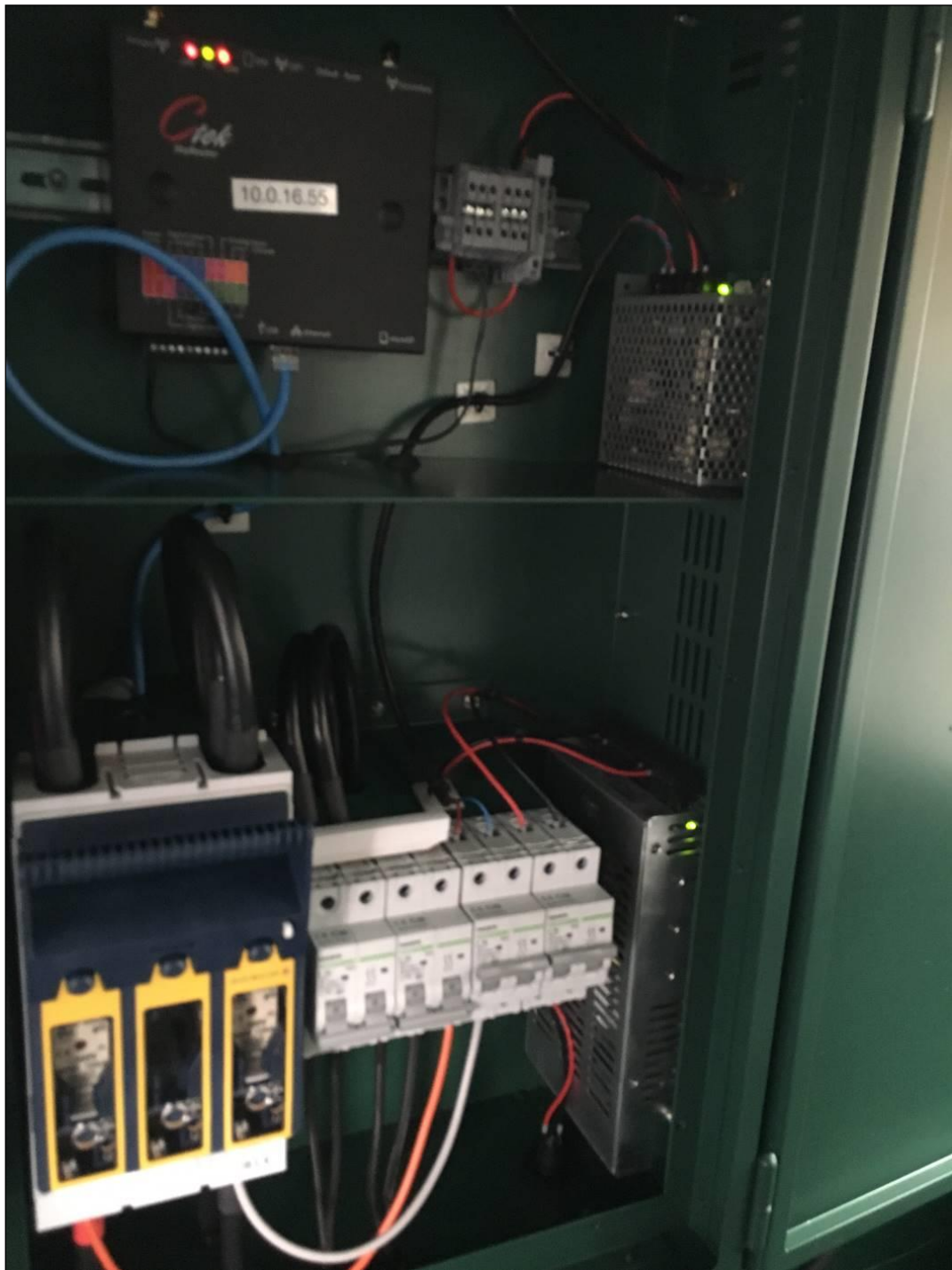
Typical Control Cabinet inside Trailer – Circuit Breakers, Fuses, and Remote Communications System
