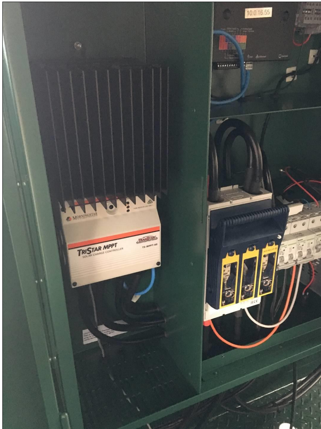
Typical Control Cabinet inside Trailer – Tristar MPPT Solar Charge Controller
